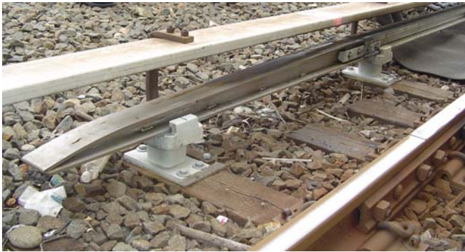
Figure 10: Fabricated End Engagement for ALSS Rail 8
