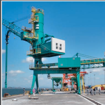
Motor Driven Cable Reel on a Ship Unloader, Korea
