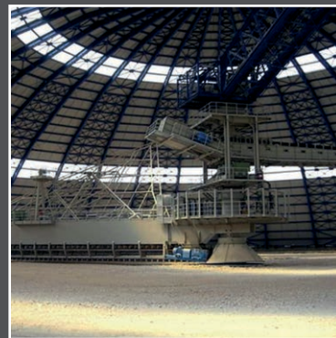
Festoon System on a Circular Bridge Reclaimers, USA
