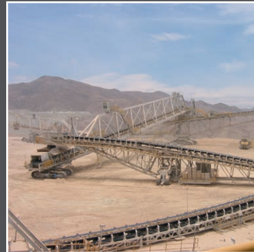
Festoon System on a Traveling Hopper, Peru
