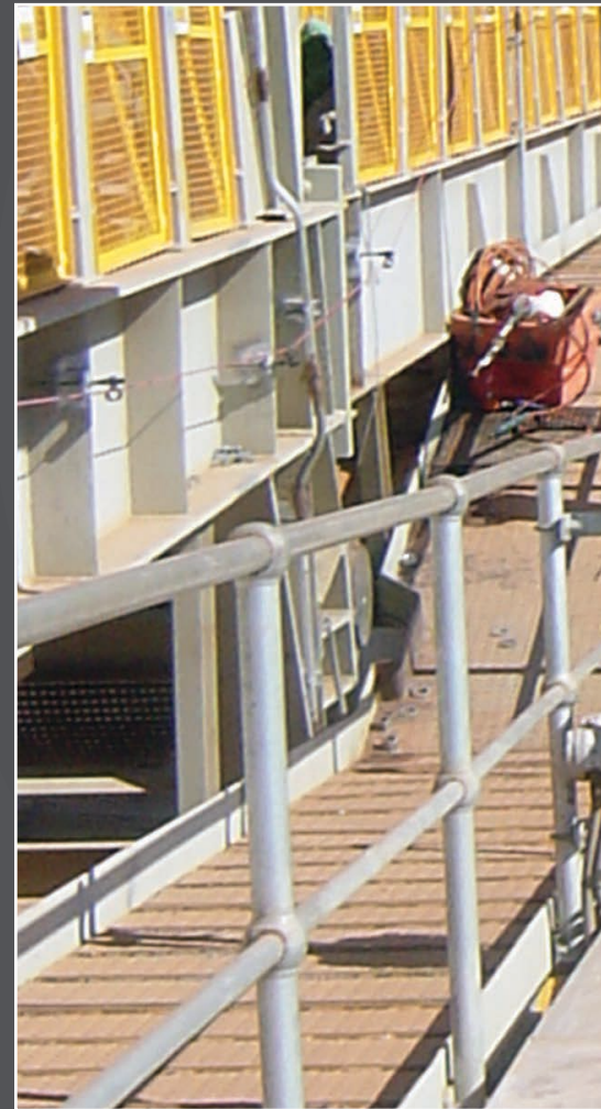
Level Wind Reels on a Stacker/Reclaimer, Australia
