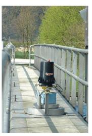
Slip ring assembly in circular scraper (sewage treatment plant)
