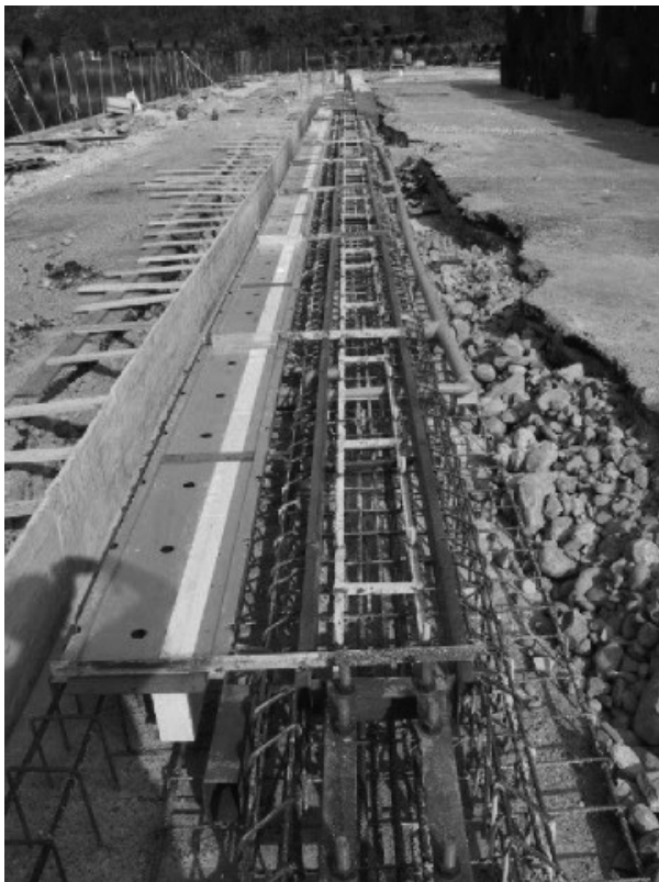
Figure 5d (above) shows site and channel system being prepared for installation.
