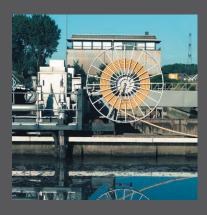
Motorized cable reel on a linear scraper bridge
