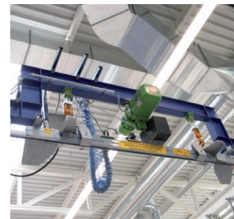
Lifting/lowering stations For bridging between different levels with a synchronous chain hoist (e.g. immersion baths or the hanging and removal of parts)
